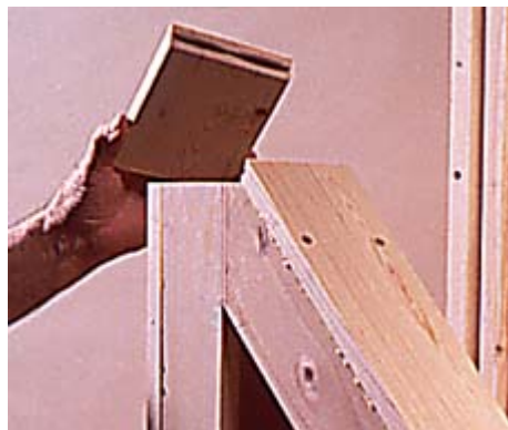
10 --After the lower case frame and back panels have been assembled, add the rails that go across the top and bottom.
