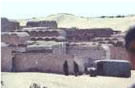
◀ Ouarglua near El Oued, S. Algeria: Single storey with efficient barrel roof vaulting in response to the absence of timber supplies
