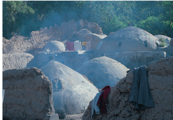
▼ Yemeni village: Domes employed for structural as well as thermal reasons. The spherical form affords progressive diurnal shading to moderate heat gain to the interior
