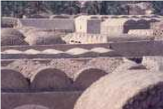
◀ Nakhla, near El Oued, Algeria: Heavily textured barrel vaulting and domes contribute significantly to the partial shading of that already provided by the curved roof forms
