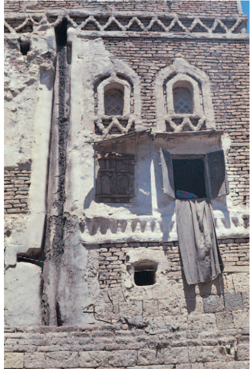
▲ Saa'na, North Yemen: The dark earthy colour is less reflective to the brilliant light and the texture provides partial shading to the surface of the building to offset solar gain
