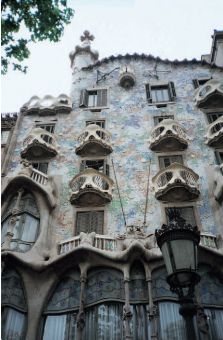
◀ Barcelona, Spain: Casa Batlló 1906, by Gaudí: The facade elements display an 'organicness'. Where the wall surface appears to be of leather, soft and supple, it glitters in numerous colours from the small round plates that project randomly like fishscales. The dreamy quality of softness and naturalness is continued inside the building
